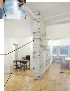
WHITE WASH EXISTING ROUGH HEWN BUILDING ELEMENTS
